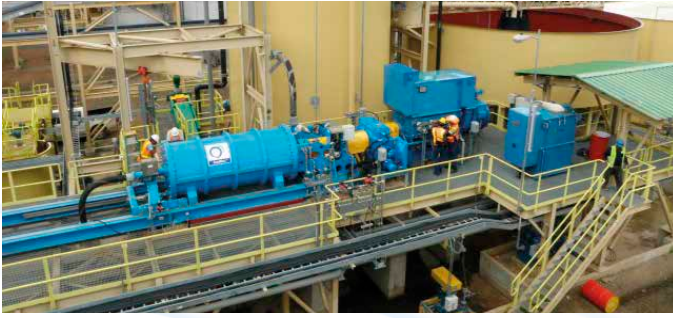
Figure 1: Las Lagunas Albian Plant
